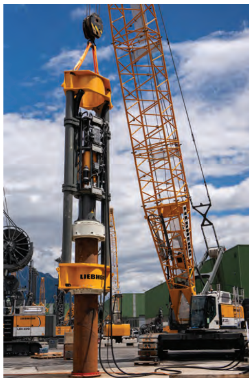
LEFT: Liebherr's rope-suspended leader with the H 10 hydraulic hammer is a cost-effective pile driving solution that can be mounted on a wide variety of cranes, including duty cycle machines, eliminating the need for a specific piling rig.
