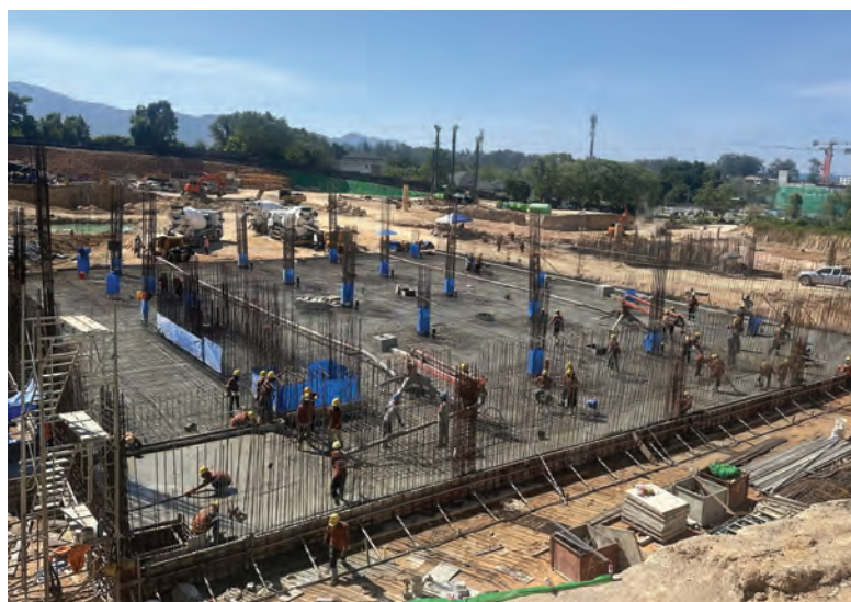
ABOVE, BELOW AND BELOW LEFT: From a construction standpoint, the challenges are substantial. The site involves extensive underground works and earthmoving operations exceeding 300,000 cu m. Elevation differences of up to 50 m across the site add further complexity to logistics, access planning and structural coordination.
