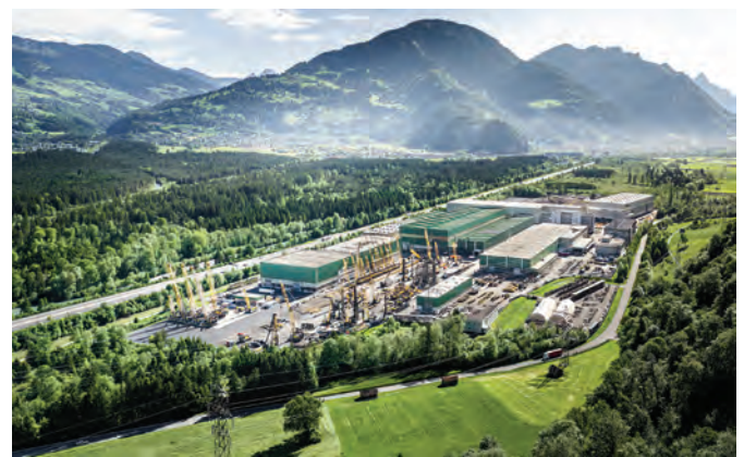
BELOW: The Nenzing site has gradually evolved from a production plant into an international innovation and competence centre.
