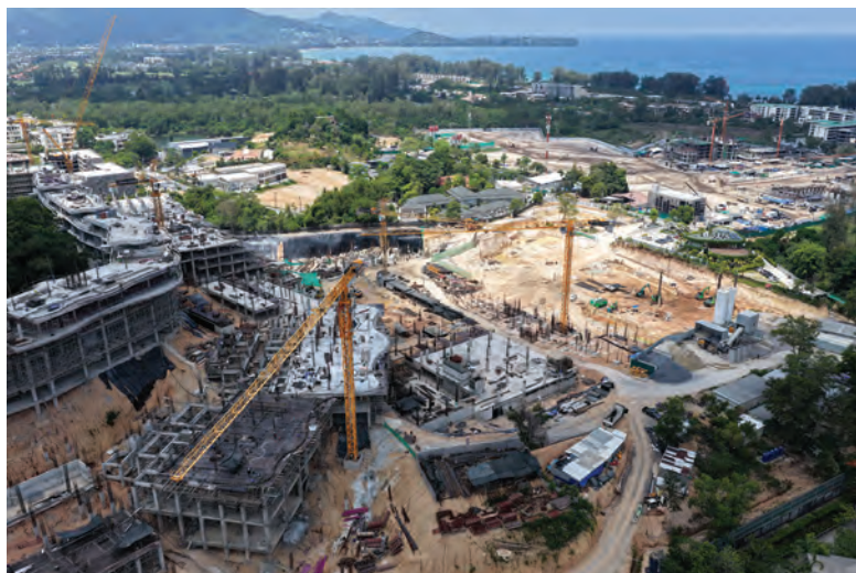
ABOVE, BELOW AND BELOW LEFT: From a construction standpoint, the challenges are substantial. The site involves extensive underground works and earthmoving operations exceeding 300,000 cu m. Elevation differences of up to 50 m across the site add further complexity to logistics, access planning and structural coordination.
