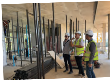
ABOVE AND RIGHT: The project team conducts site inspections. With the developer-led delivery approach, key coordination issues are typically resolved within a 48-hour timeframe, allowing construction activities to progress without prolonged delays in decision-making.
