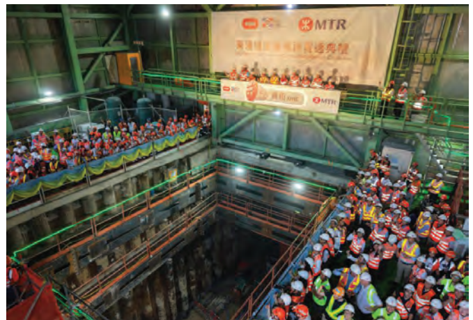
TOP AND ABOVE: The tunnelling breakthrough ceremony for the Tung Chung West section was held on 22 June 2026.
